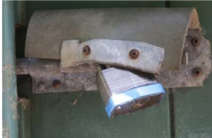
Leather, vinyl, or rubber tarp can be affixed over the top of the shackle
